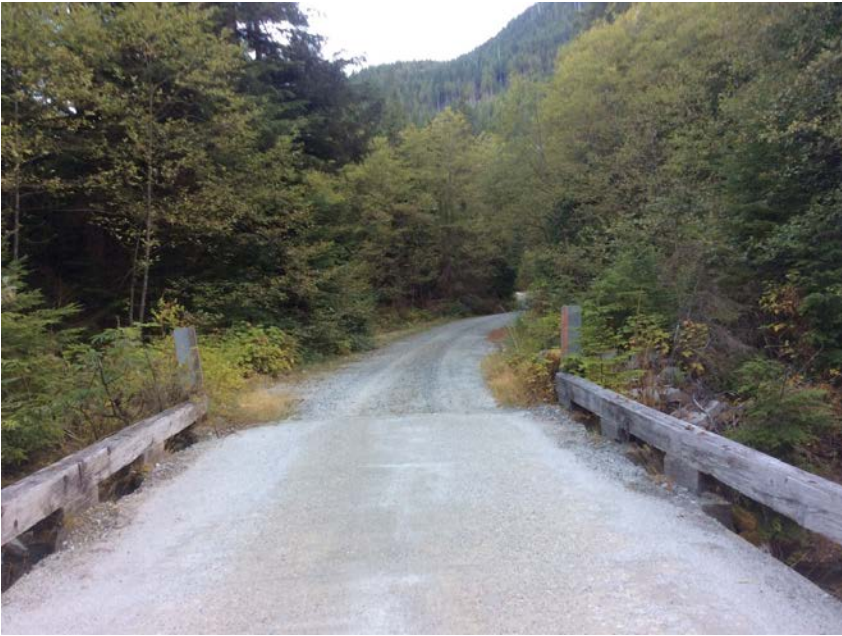
Right approach viewed from bridge
