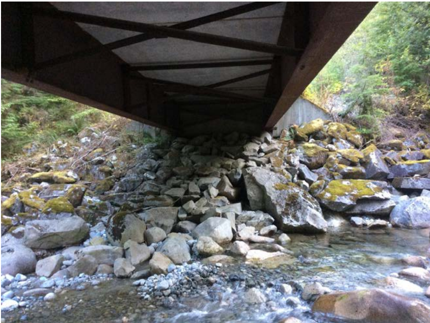
Right Bank Abutment when facing downstream
