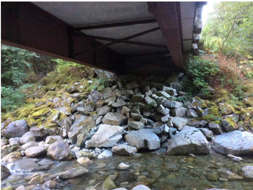
Left Bank Abutment when facing downstream
