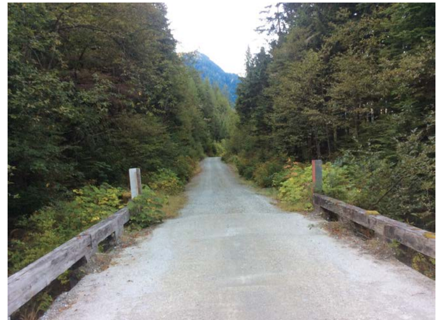
Left approach viewed from bridge
